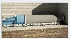
After the auger arrives at the end, the rotation movement stops. The machine is withdrawn by the pipe length, and the other pipe which has an auger in is lowered. By welding, this
