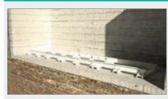
The walking rails of the machine are located in the chimney by a crane, and are located on the base concrete. The walking rails are adjusted according to the drilling axle. The middle axle of the rail should match with the drilling axle.
