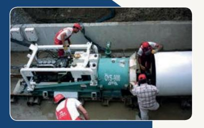
Özkanlar Horizontal Thrust Boring Machines are designed to bore the inevitable need of many public works and construction applications, the coated holes of diameter between 12" and 120".
