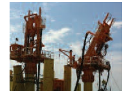
RCD R1820 Malaka Gas Terminal, West Malaysia
