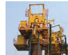
RCD R3030 Hyomyong-Myungji Bridge, Korea
