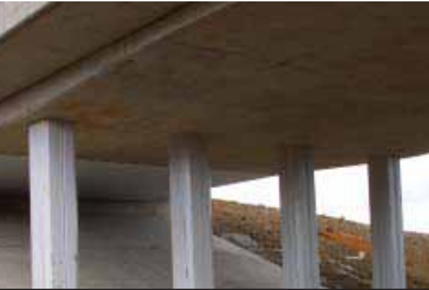
Structures are designed and built for shorter working lives. The cycle of re-construction comes round faster
